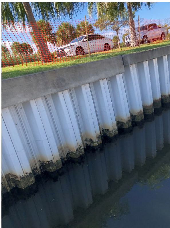
Photo #10 – View of Seawall Cap Change and Cap (Right Cap in Photo) Alignment Out 4 Inches
