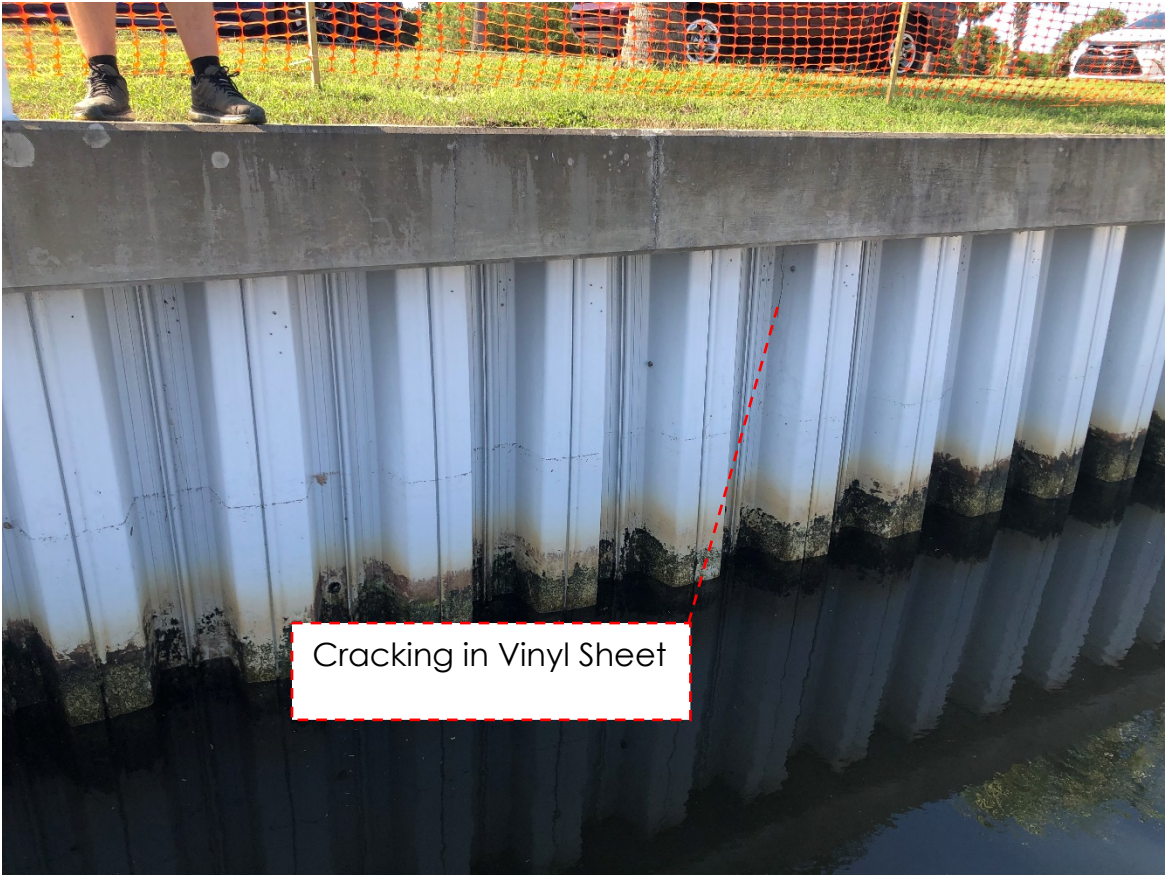
Photo #12 – View of Horizontal Cracking in Seawall Cap
