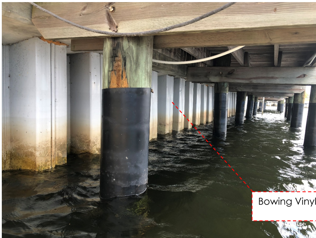
Photo #16 – View of Bowing Vinyl Sheets Underneath Docks
