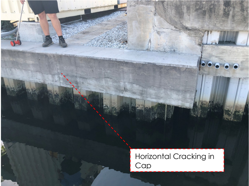
Photo #12 – View of Horizontal Cracking in Seawall Cap
