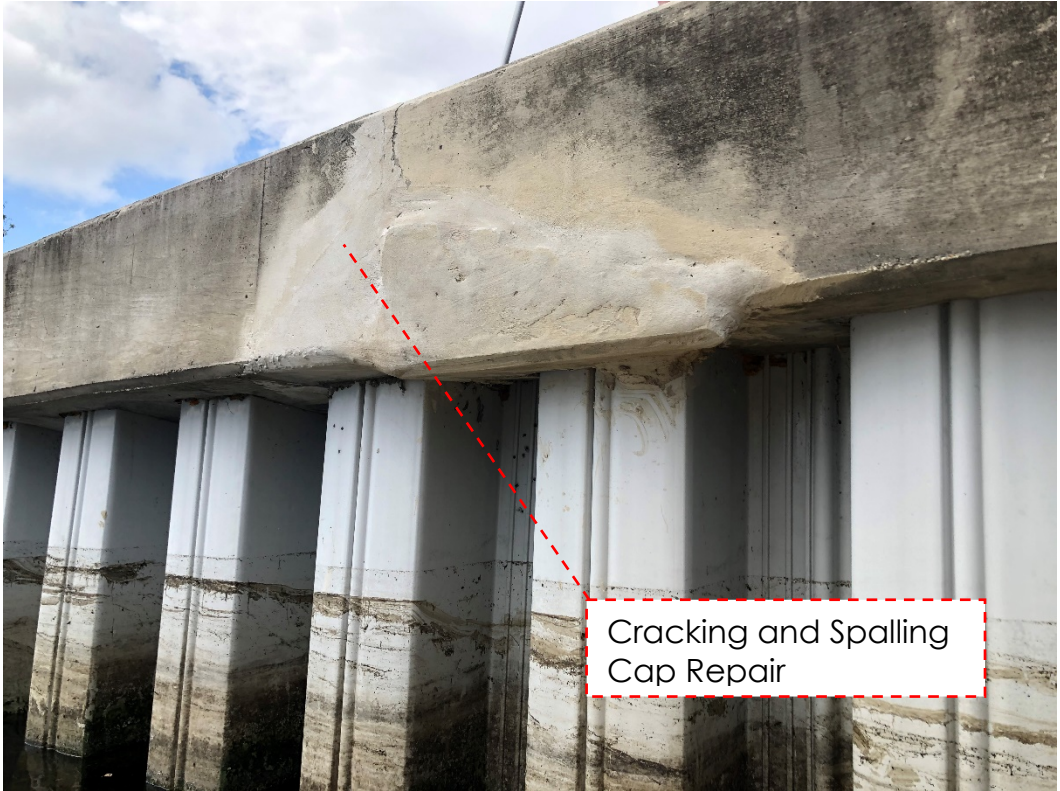
Photo #18 – Repaired Section of Spalling in Cap
